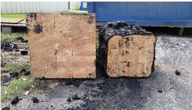
Figure 14: Fire-resistance ratings can impact required member size. Shown here are glulam columns, pre- and post- 2-hour fire test. Source: David Barber, ARUP
