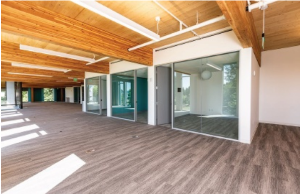
Figure 6: First Tech Credit Union, Hillsboro, OR. 12x32-ft grid with 5.5-in. CLT panels spanning 12 ft between glulam beams. Source: Swinerton Mass Timber.
