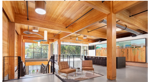
Figure 1: DPR Construction Headquarters Office Building, Sacramento, CA. CLT and glulam construction. Source: SmithGroup, Buehler Engineering; photo Chad Davies
