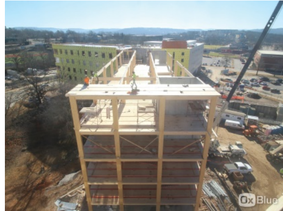
Figure 11: Adohi Hall, University of Arkansas, Fayetteville, AR. 20-ft grid increments maximized 40-ft long CLT panels for minimal waste. Source: Leers Weinzapfel Associates, OxBlue
