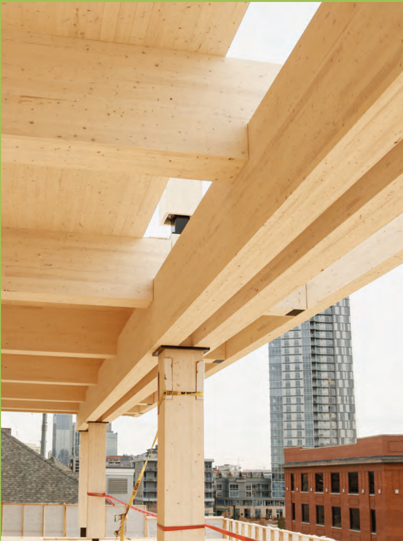
Glulam columns and beams supporting CLT roof panels
