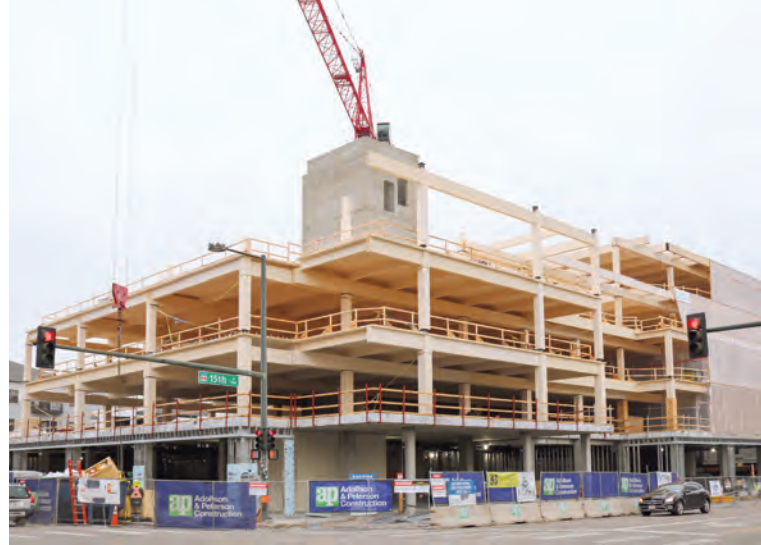
Mass timber reduced construction time by 20%
