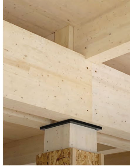
Column connected to CLT beam and girder
