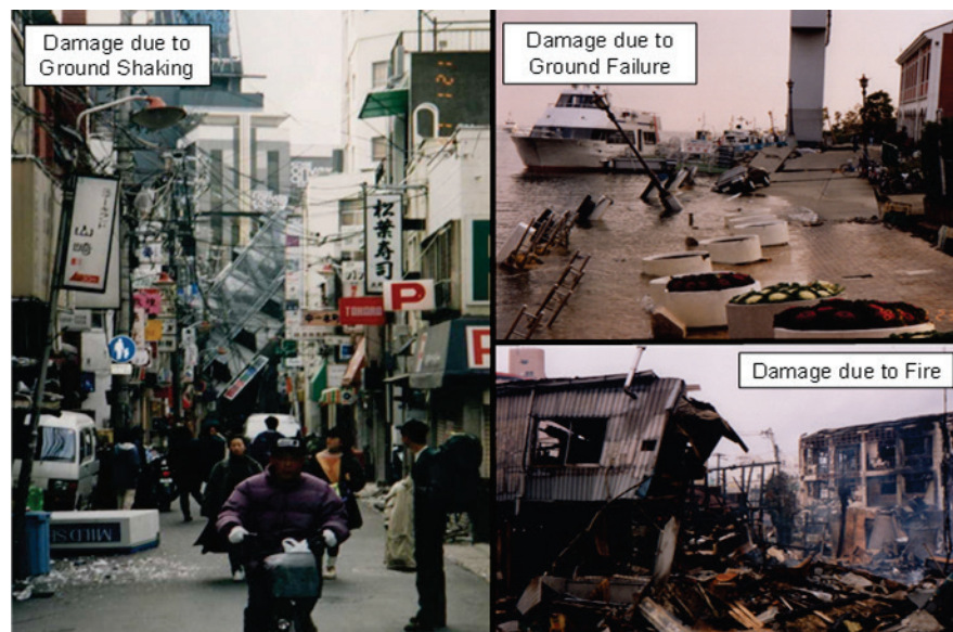
Figure 2-11 Typical street scene in Kobe City immediately after the earthquake; damage at a ferry terminal due to ground failure (liquefaction); and a neighborhood destroyed by fire.
