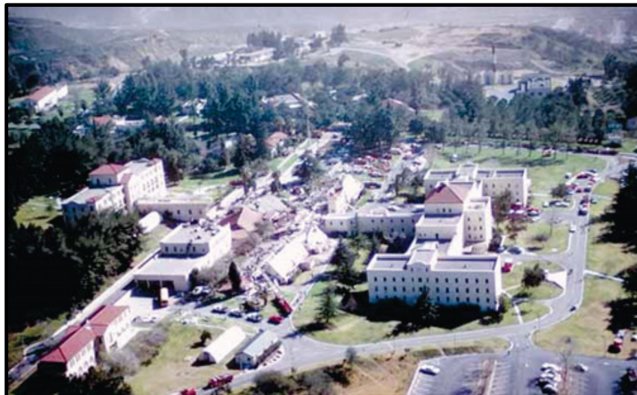
Figure 2-2 Collapse of non-ductile concrete frame buildings at the Veterans Administration (VA) complex in the 1971 San Fernando earthquake.
