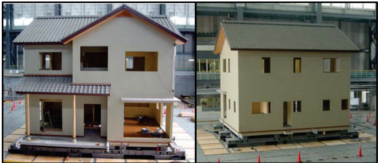
Figure 2-15 Test building on the E-Defense shake table prior to testing, showing views of the front (left) and back (right) of the test building (Isoda et al., 2008).
