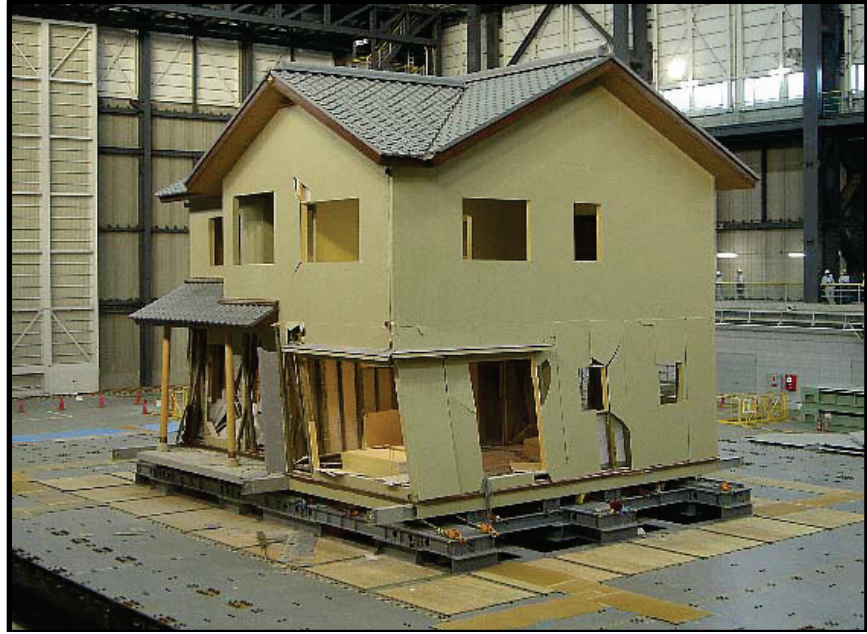
Figure 2-17 Severe first-story damage and leaning of the test building after the second JR Takatori shake (Isoda et al., 2008).
