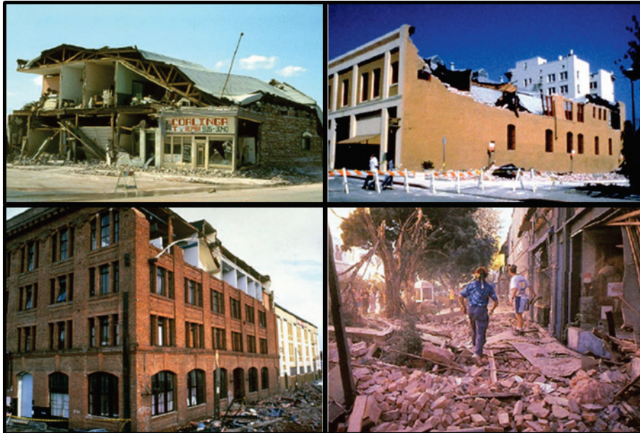
Figure 2-1 Collapse of URM buildings in the 1983 Coalinga earthquake (top left), the 1987 Whittier earthquake (top right), and the 1987 Loma Prieta earthquake (bottom).
