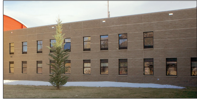
Figure 2-7. Perforated wall (low-rise office or school).
