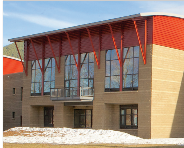
Figure 2-8. Coupled wall with beam coupling (school).
