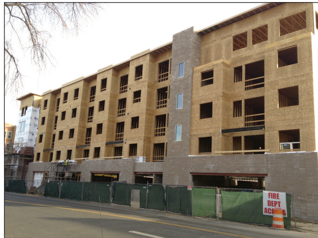
Figure 2-6. Cantilever wall (residential with light wood framing).
