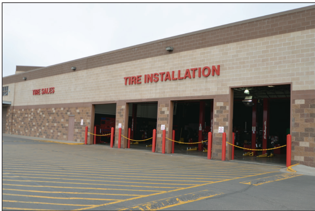
Figure 2-5. Line of resistance with disparate wall stiffnesses (typical of low-rise retail and industrial buildings).
