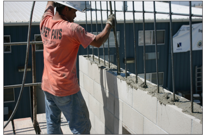
Figure 7-4. Consolidation of grout using a vibrator.
