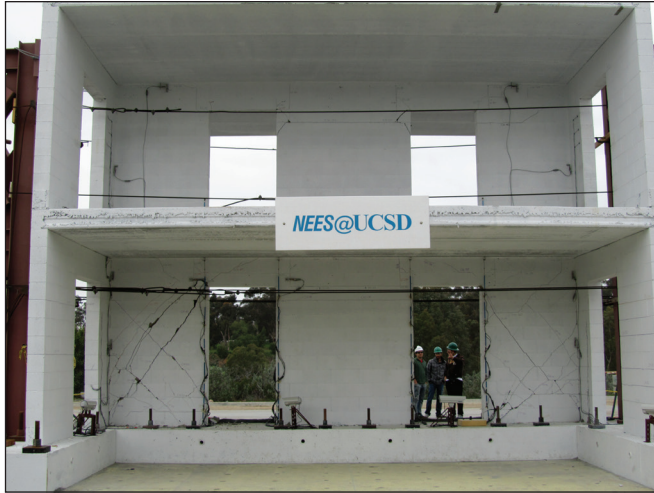
Figure 3-8. Shear failure of reinforced masonry walls in the first story during a shake table test.
