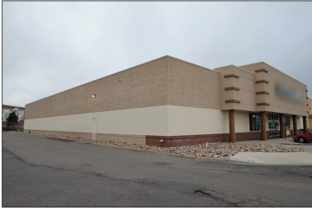
Figure 2-4. Squat, shear-dominated wall (typical of low-rise retail).
