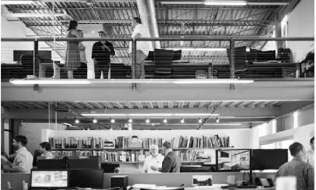
The Freight Building in Denver, Colorado showing the new structural steel floor and old open web joists used for the new roof. KL&A performed the structural engineering.
